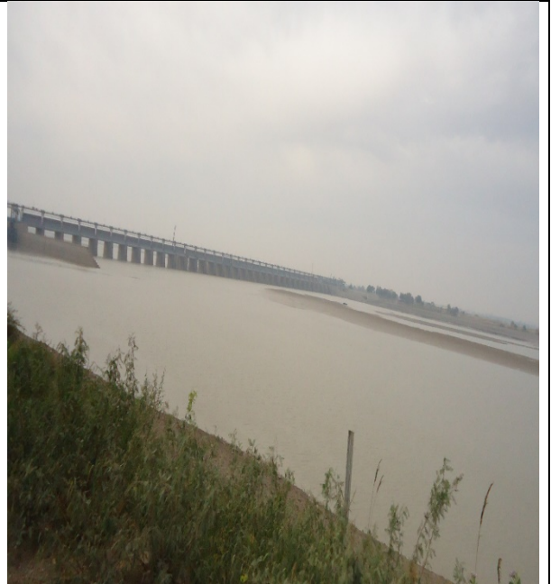
Pic 2: Barrage at River side of Bund
