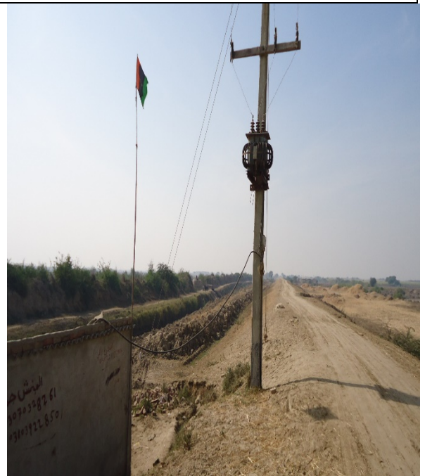
Pic 4: Electric Poll at Land side of Bund
