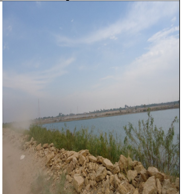
Pic 4: Water at Land side of Bund
