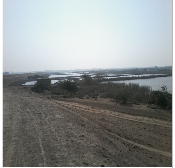
Pic 2: Land side of Bund
