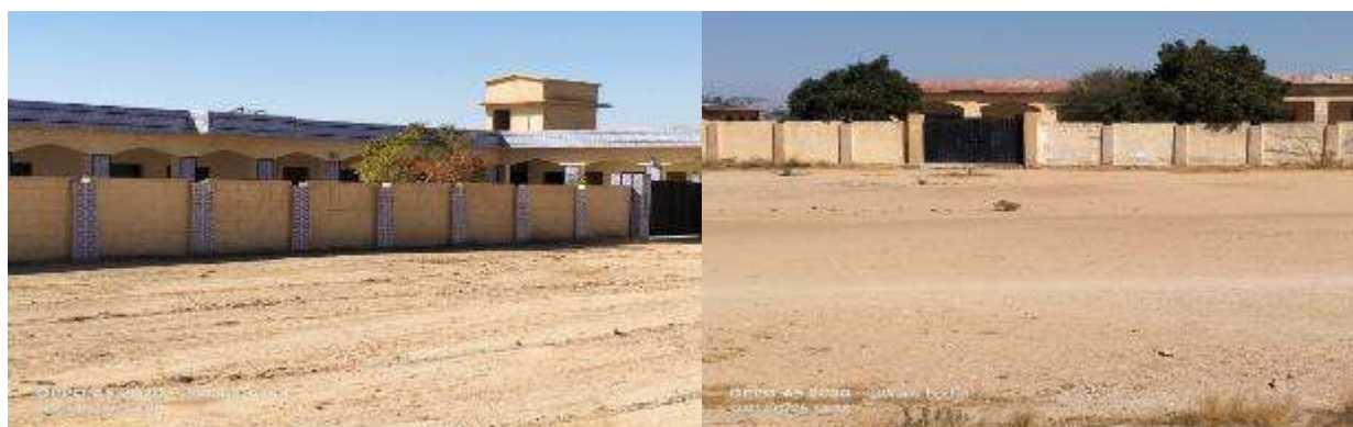
Figure 19: Boys Middle & Girls Primary School at Sub-Project Area
