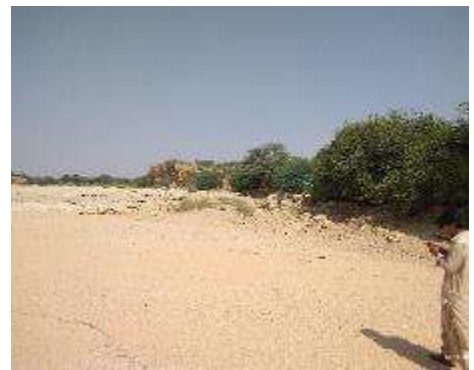
Topography of proposed Asabo dam site
