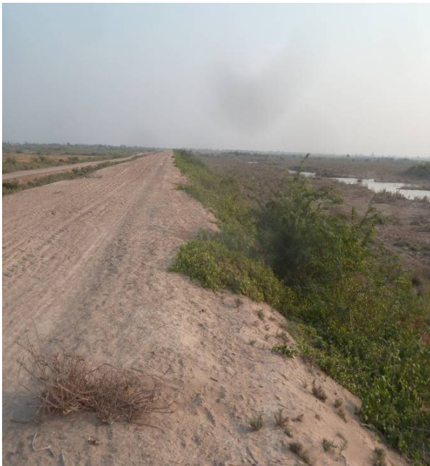
Picture 3: View of MS bund (River Side)
