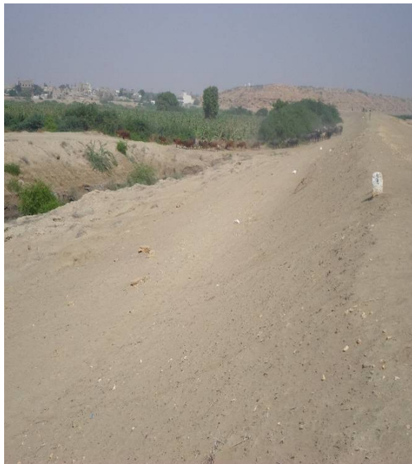
Picture 3: View of SH Bund (Land side)
