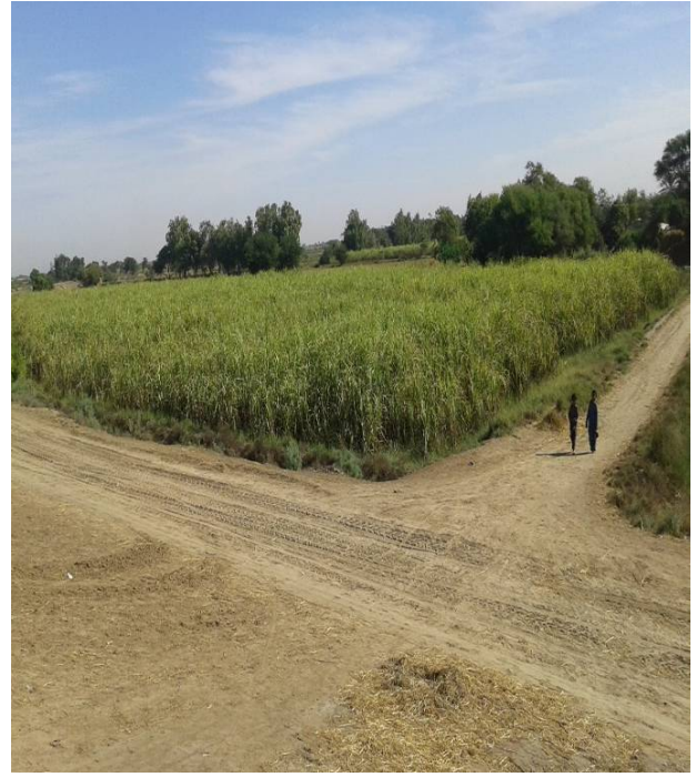
Picture 2: View of MS bund (Land side)
