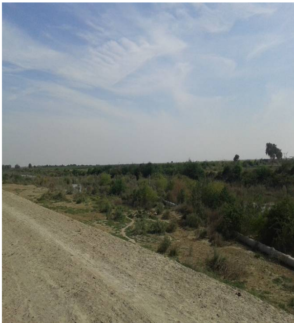
Picture 3: View of BU Bund (River Side)
