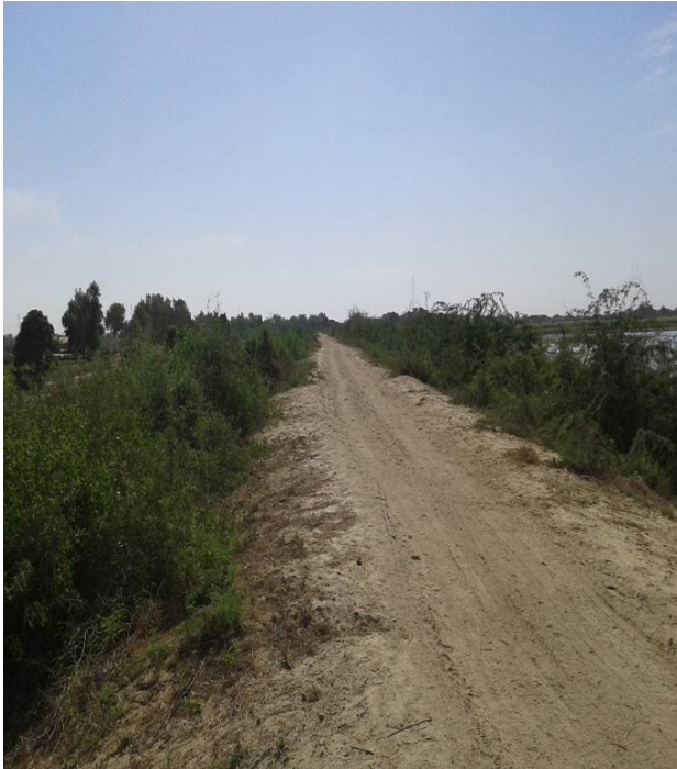
Picture 1: View of MS bund
