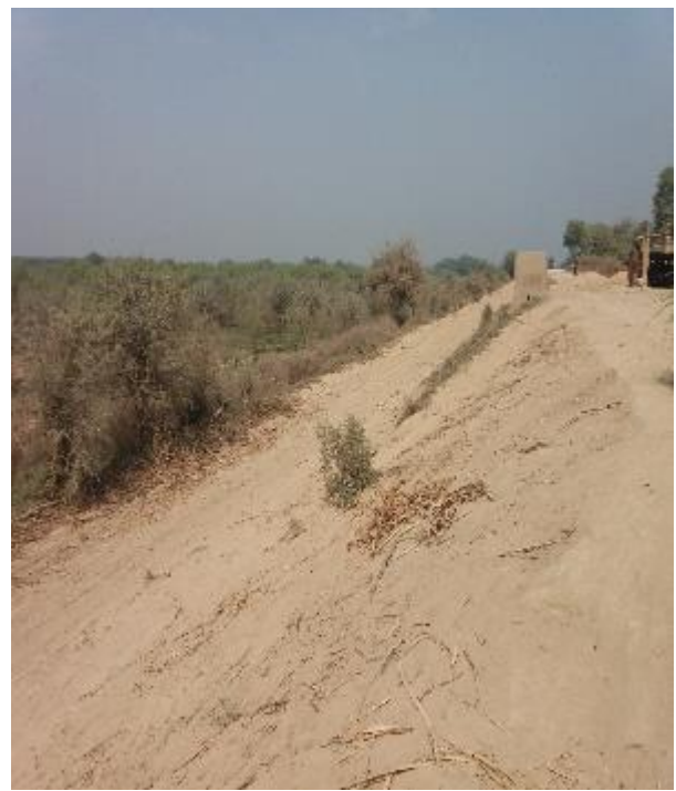
Condition of Community Ramp at 124/2
