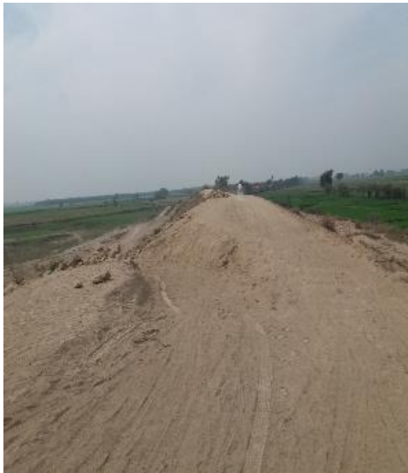
Existing Condition of embankment at 154/4
