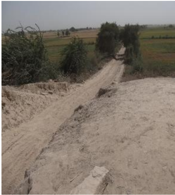
Ramp at 150/2 inner side
