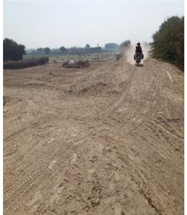
Existing condition of embankment at 168/0
