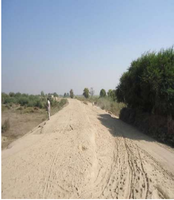
Pre-project View of M.S Bund
