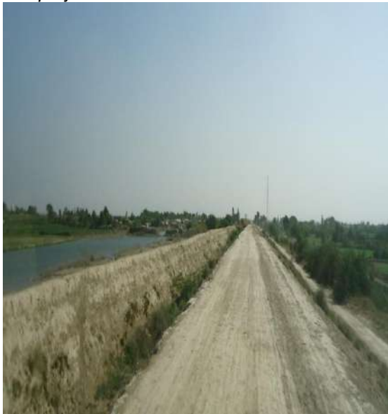
Pre-project Condition of B.U Bund
