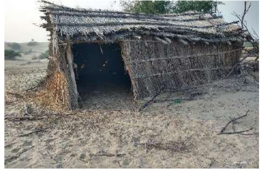
Type of construction at Khurrand site
