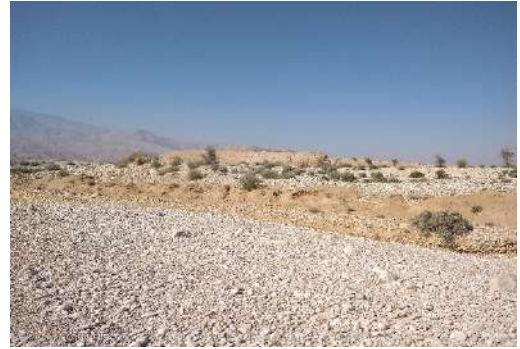
Topography of Narani Dam site
