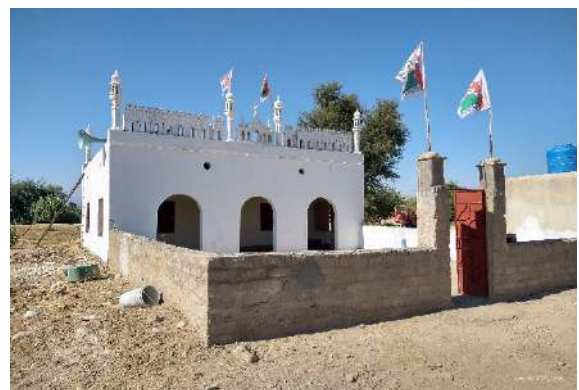
Mosque at Khinji Dam Site Area
