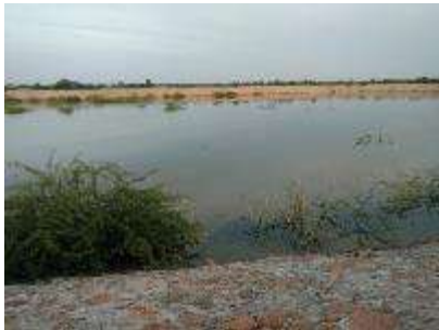
Pond a sub project area
