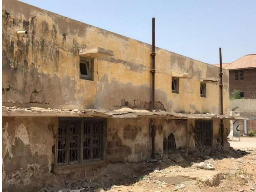
Figure D.1: Existing Condition of Soil Mechanics Laboratory Karachi
