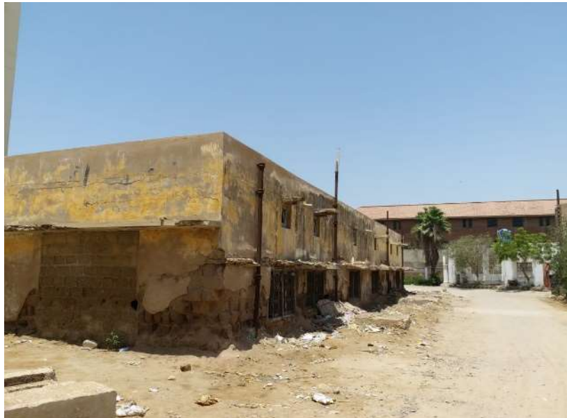
Figure D.2: Another view of existing building of Soil Mechanics Laboratory
