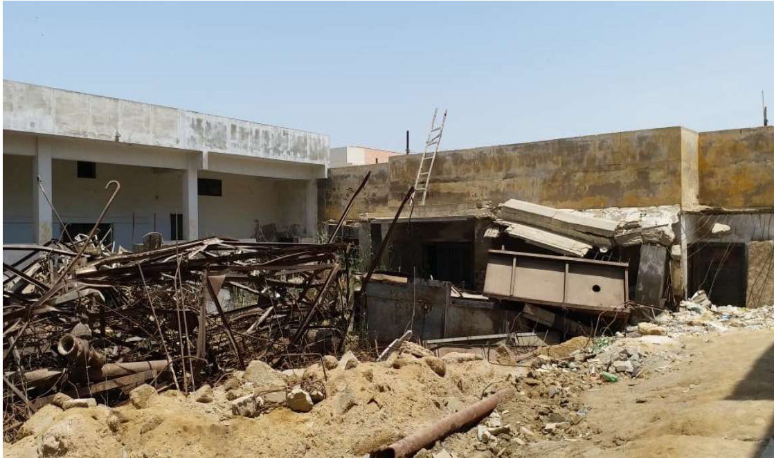
Figure 4: Another view of existing conditions of Soil Mechanics Laboratory
