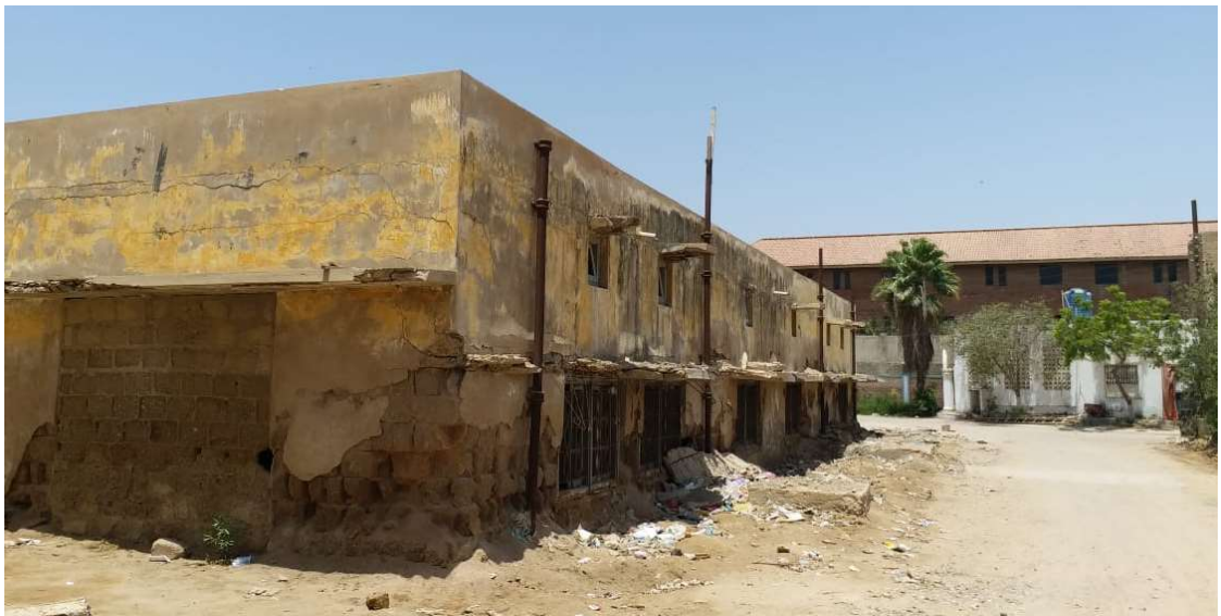
Figure 3: Existing conditions of Soil Mechanics Laboratory
