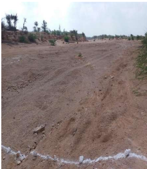
A View of Karmatiani Dam Site
