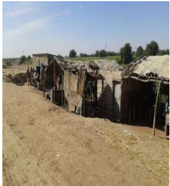
Shops and tea stall at MS Bund 49.4 (River side)
