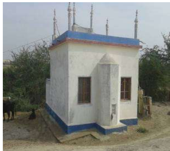
Mosque at MS bund 37.25 Mile (Community Side)
