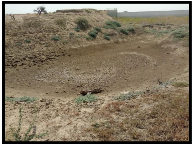
Dry pond (Taraee) at Sabusan Dam
