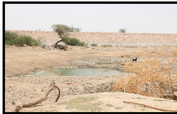
Excavated Pond Inside Sankar Dam
